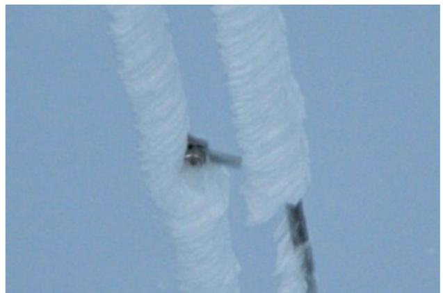
Fig. 16. In-cloud icing on duplex conductor in FL4 (400 kV OHTL) in Dec. 2006.
