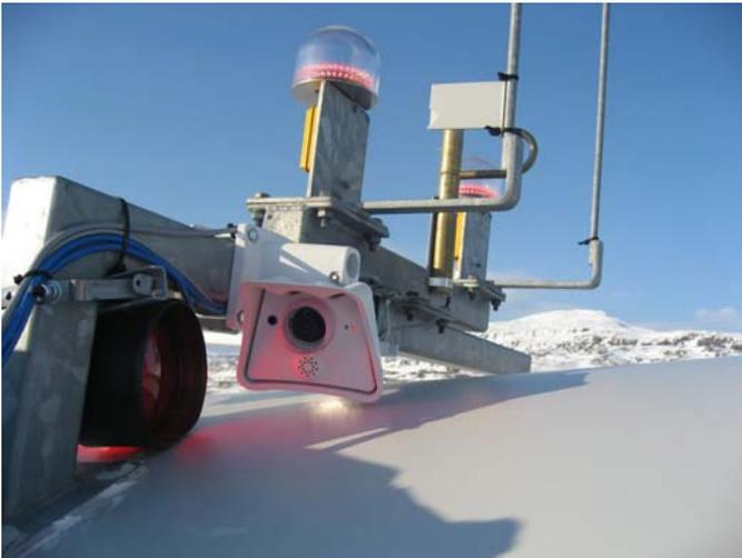
Figure 2: Web camera mounted on light boom.
