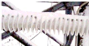
Long rod insulator, horizontal set-up
