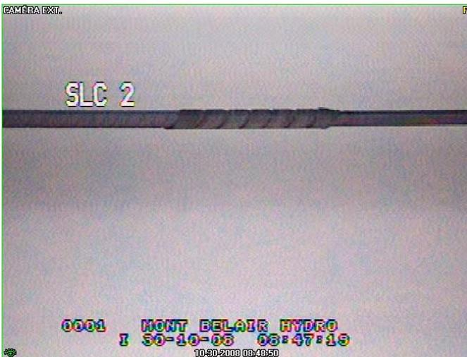
Fig. 15. Junction of single-layer and double-layer LC-Spiral Rods.
