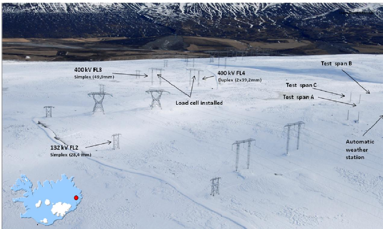
Fig. 1. Hallormsstadahals, measuring site with 3 test spans and measurement in two suspension towers in 400 kV OHTLs.
