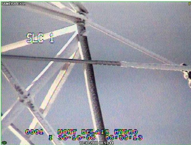
Fig. 14. Right-hand extremity of LC-Spiral Rods with end rods and vibration damper.
