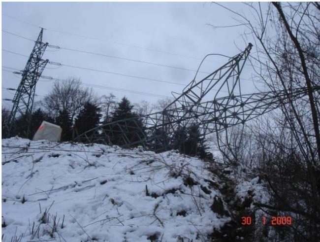
Fig.9: One of collapsed towers
