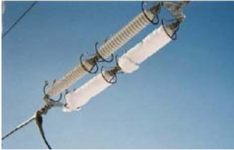
Fig.1 Example of packed snow on horizontally mounted long rod insulator strings.
