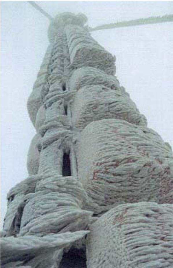
Fig. 2. Photograph of icing accumulated on Kivenlahti TV tower (courtesy of A. Photographer).
