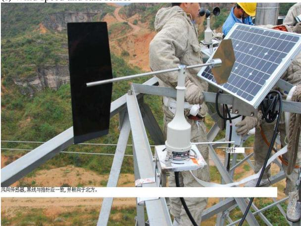
(g) wind direction sensor and solar bar
