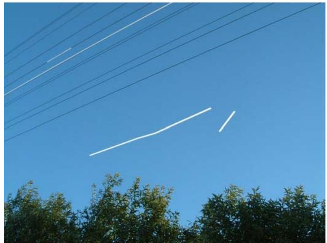
Fig. 1. Chunks of snow falling from an overhead transmission line.
