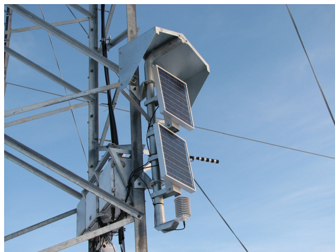
Fig. 12. Monitoring equipment in a 400 kV line.
