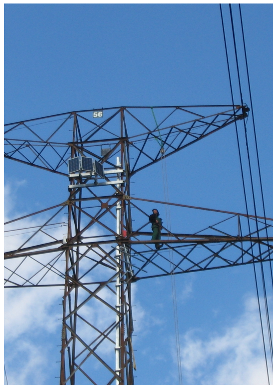
Fig. 4. Solar panels at the top of the tower on line 400 kV (location Nosovice)
