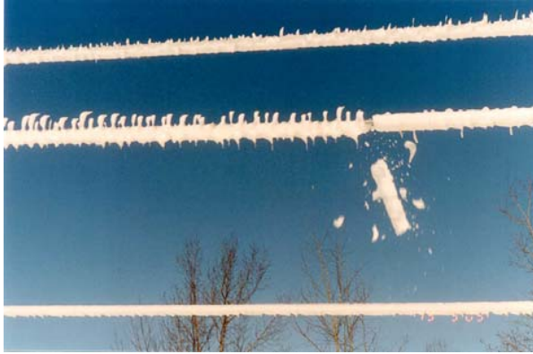
Photo 3 Ice deposits sliding and shocking in the middle of the span
