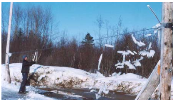
Photo 11 Complete de-icing in less than a full turn
