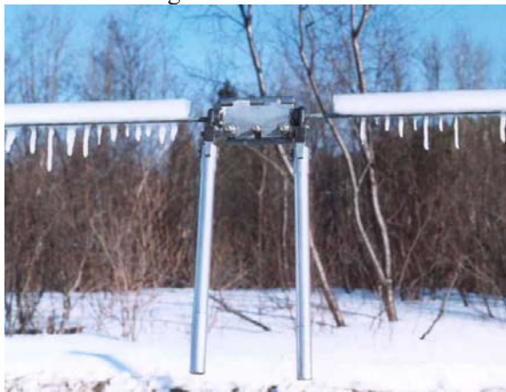
Photo 9 Twisting device fully installed with two handles
