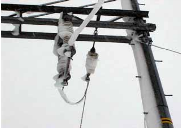
Fig.6 Transmission pole and insulators covered with snow after snow storm
