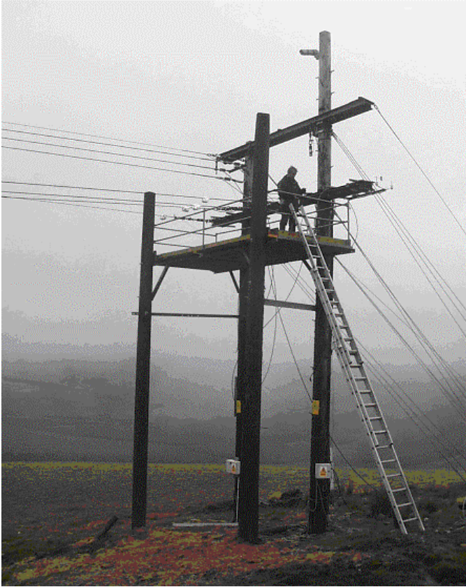
Fig. 2.1 The access platform at the southern H-pole
