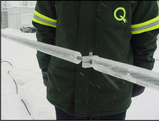
Fig. 12. Accelerometer installed on the GW with concentric ice accretion.
