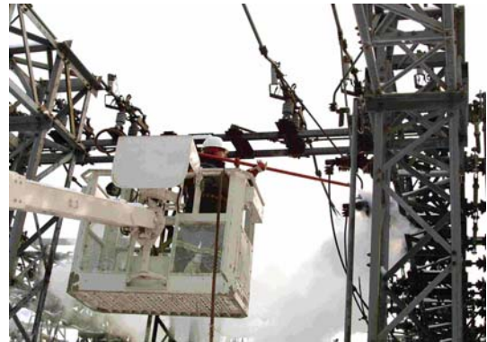
Figure 4a: Steam cleaning
