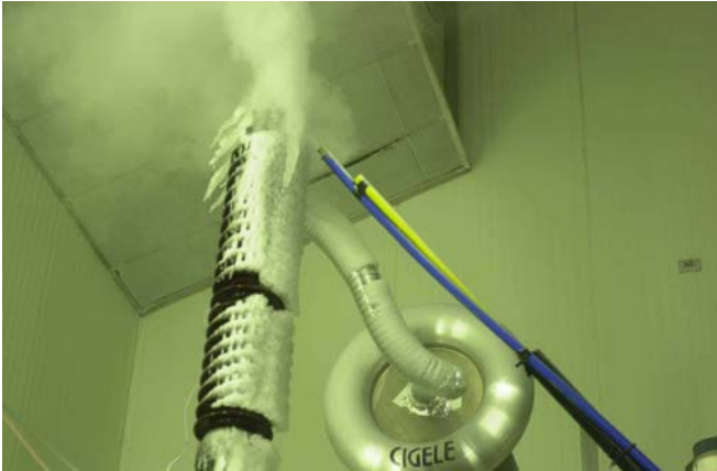
Figure 3: De-icing test on the jaw of an energized disconnect switch.
