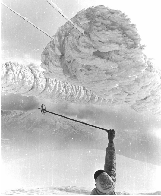
Fig. 1. Rime icing on a 22 kV line on Lønahorgi, 1 400 m asl, near Voss, Norway, April 1961. (Photo: O. Whist)
