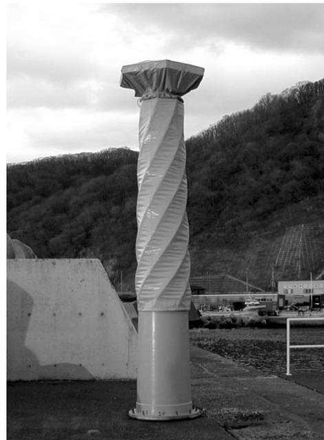
Figure 8 FRP lighthouse wrapped by membrane structure.
