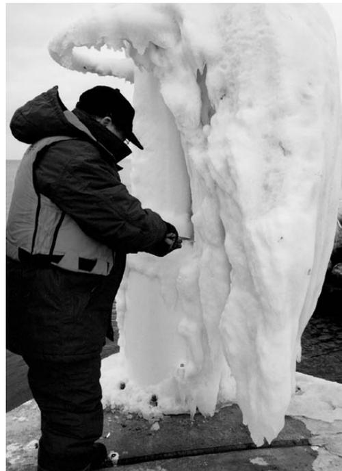
Fig. 1. Sea spray icing on a small lighthouse.
