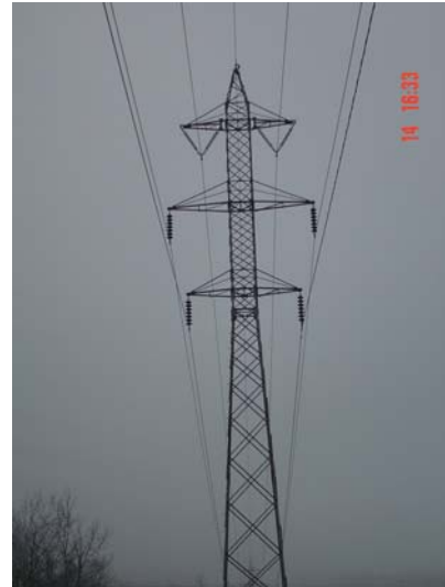
Fig. 5: Suspension tower after modification.
