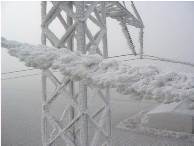
Fig. 3. Example of build-up of low density ice accretion on conductors
