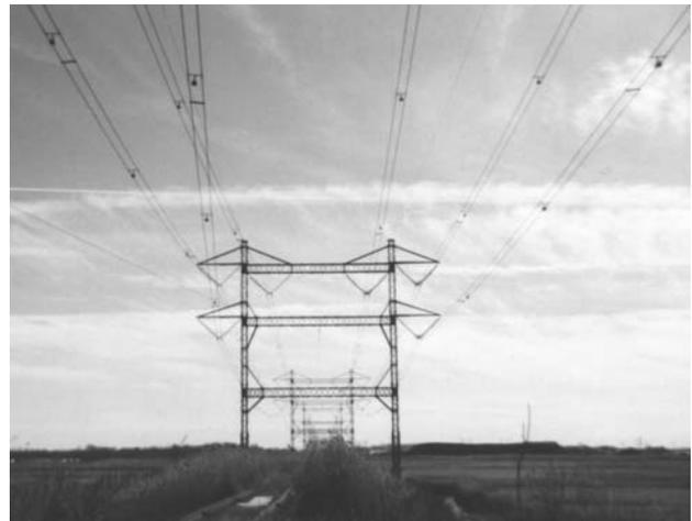
Fig. 6. Detuning pendulums for galloping control installed on a 345 kV line.
