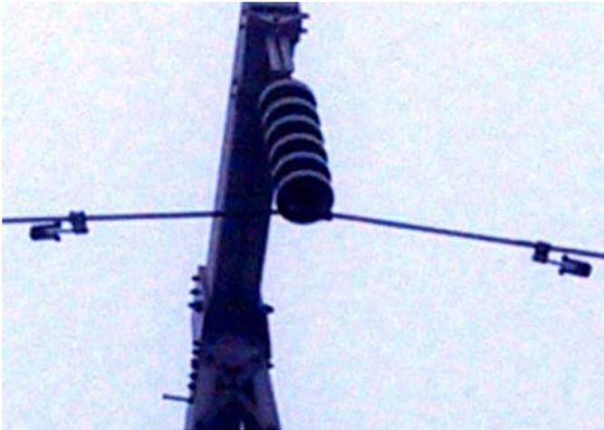
Fig. 1: Stockbridge dampers with missing masses on a transmission line
