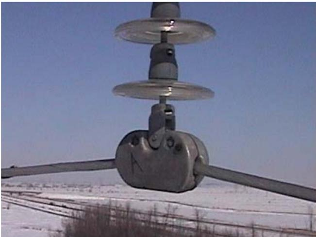
Fig. 9: Metal-to-metal clamp
