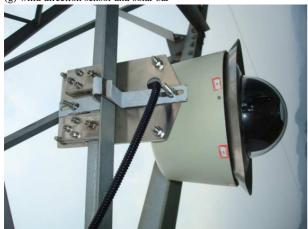
(h) Video Fig.3 Installation of online monitoring unit
