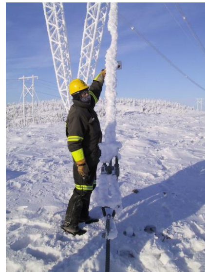
Figure 2. Detail of rime accretion on support cable
