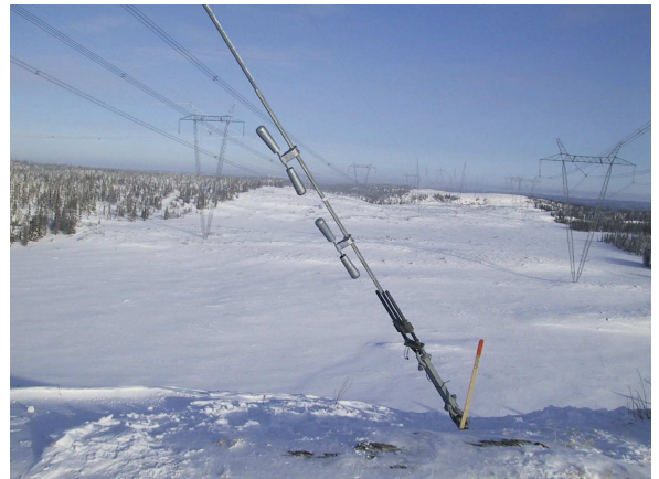
Figure 3: Dampers installed on guy support cables (James Bay 735 kV network)
