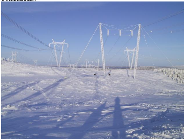
Figure 1. Hard rime accretion on James Bay transmission network
