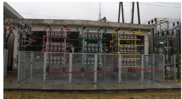
Fig.3 Regulative Capacitor Series—Wound Compensate AC De—Icer
