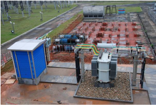
Fig.5 Fixed DC De—Icing Device
