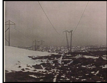
Figure 7: Bridge Failure at the top of Hawke Hill (Haldar, 2007)
