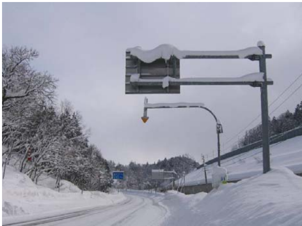
Figure 1. Example of snow accumulation on road information sign.
