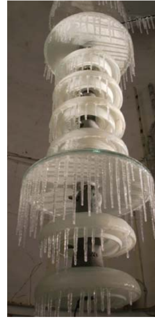
Figure 3. The icing insulators of “4+1” insulator strings with alternating diameter sheds
