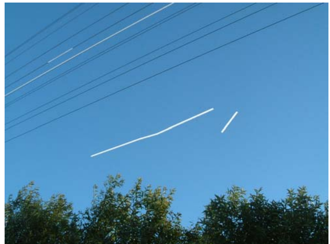
Figure 1. Chunks of snow falling from an overhead transmission line.
