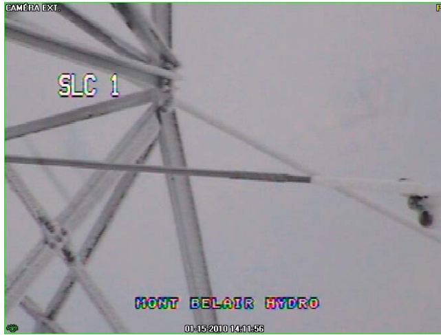
Figure 6. Photo taken from the remote-control camera showing the right-hand extremity of LC-Spiral Rods with end rods and vibration damper.
