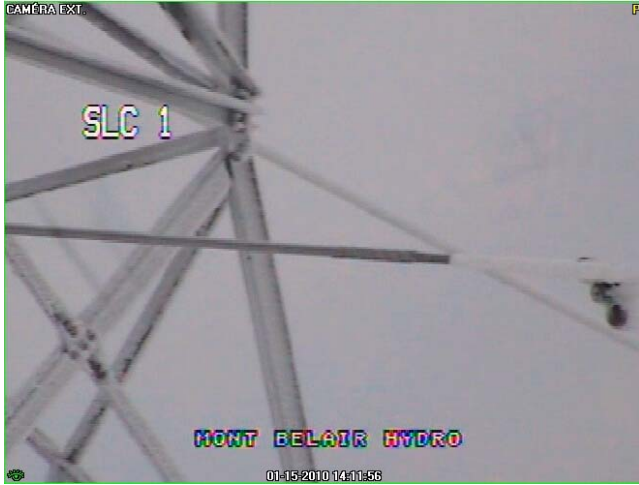
Figure 6. Photo taken from the remote-control camera showing the right-hand extremity of LC-Spiral Rods with end rods and vibration damper.
